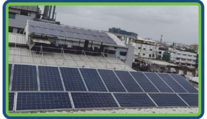
100 Kwp Rooftop Solar System Installation & Commissioning At Dharmanandan Diamond, Katargam, Surat
