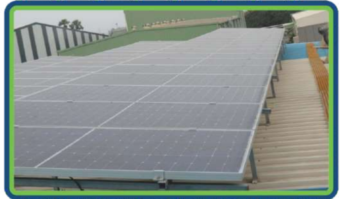
270Kwp Rooftop Solar System Installation & Commissioning At Anand International, Bhatpore, Surat
