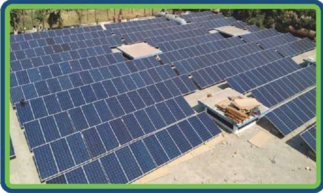
200Kwp Groundmounted Solar System Installation & Commissioning At SMC, puna, Surat
