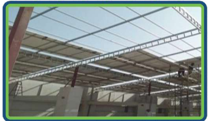
125 Kwp Rooftop Solar System Installation & Commissioning At Milenium-2
